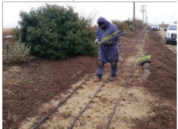
FIGURE 4.15: In some areas, such as California, irrigation may be necessary to establish new wildflower plantings from seed and should be included in the planning and installation phases of a project.
